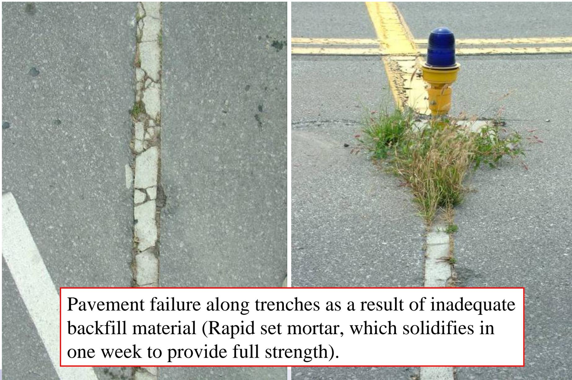
Pavement failure along trenches as a result of inadequate backfill material (Rapid set mortar, which solidifies in one week to provide full strength).
